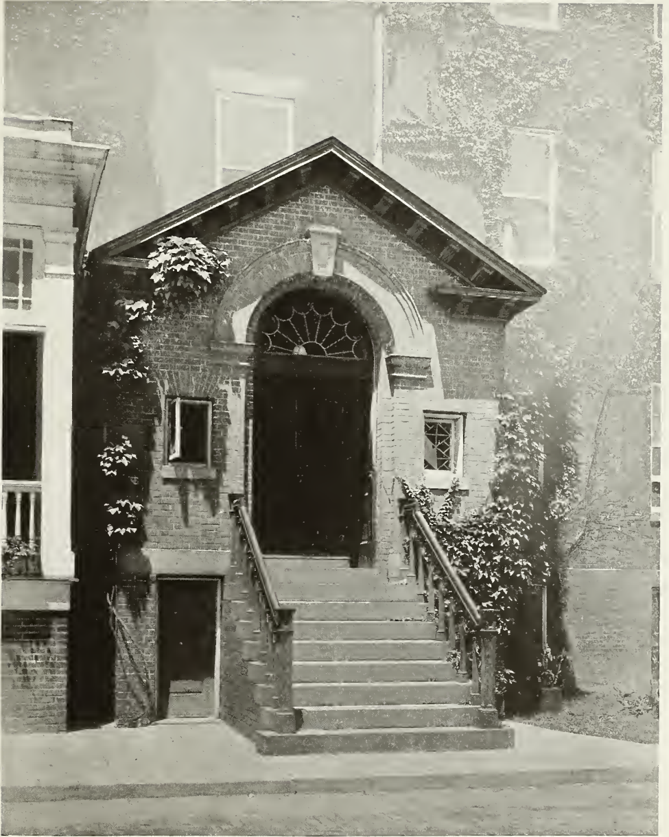
THE FRONT DOOR LEADING TO THE OFFICE
